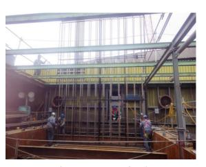
Installing RDE and its frame
